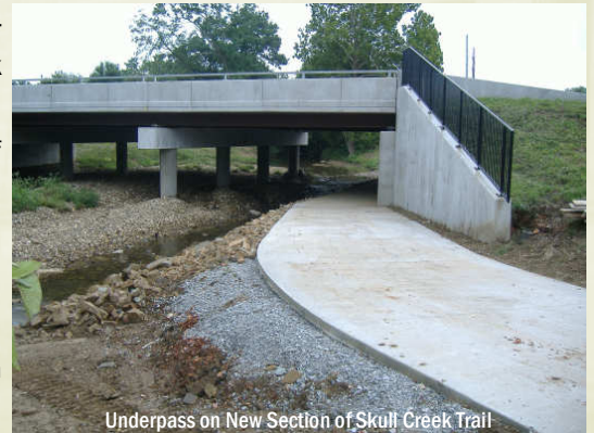
Underpass on New Section of Skull Creek Trail
